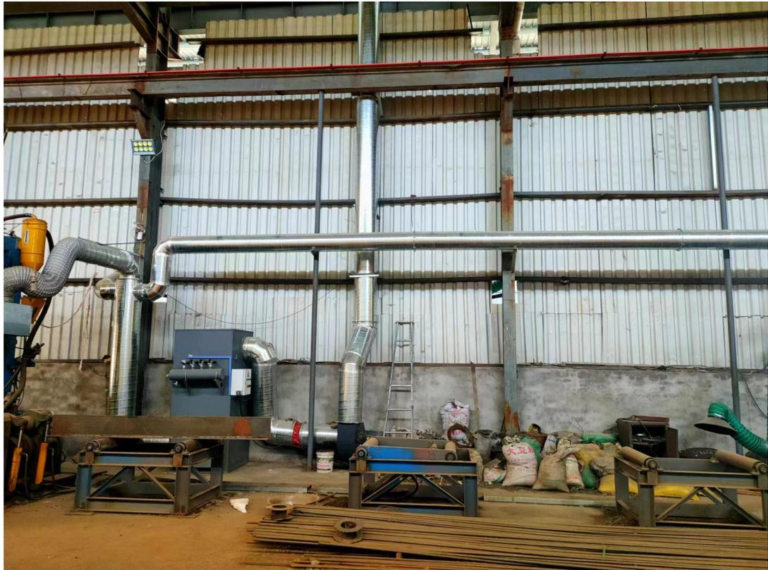
焊接工序焊烟净化器+15米排气筒
